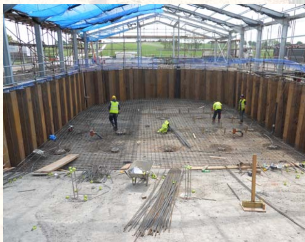
Week 12: the shell is up and the recess complete
