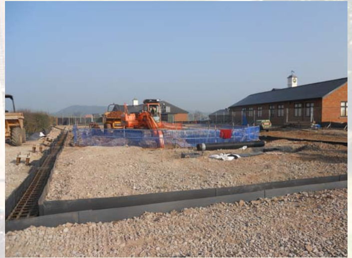
Week 7: foundations in and pool being dug out
