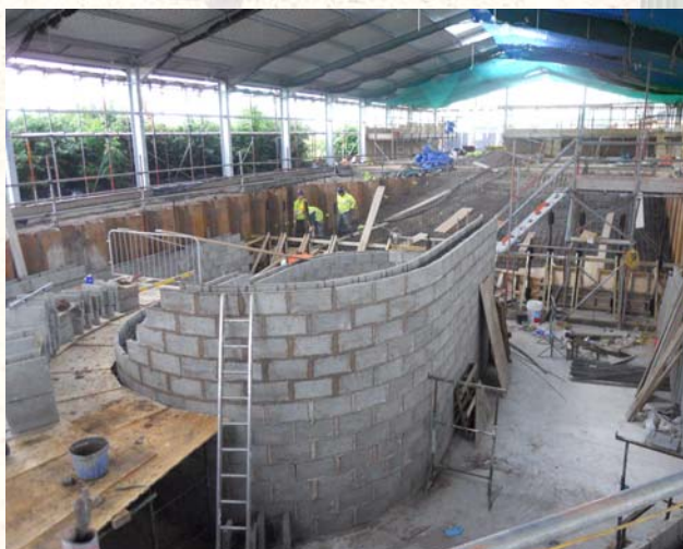
Week 16: Pool walls & island nearing completion
